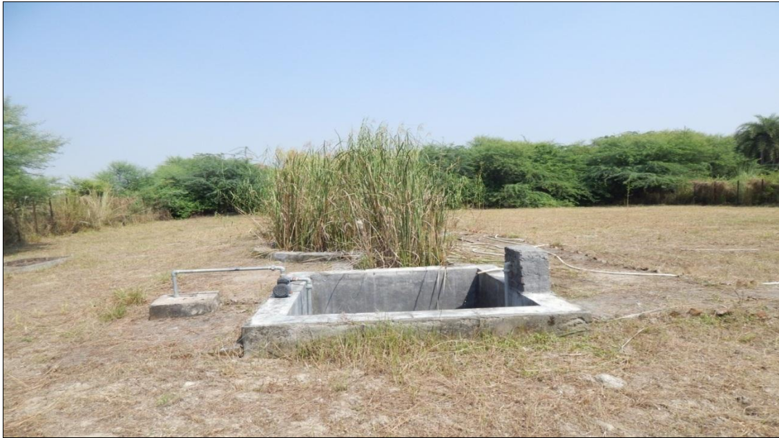
Fig 9.2: Designed pilot plant with constructed wetland plant treatment system with Phragmites communis and Typha latifolia
