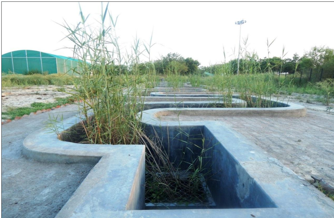
Fig 9.3: Luxuriant growth of Phragmites communis and Typha latifolia in designed constructed wetland treatment system for detoxification of Post Methanated Distillery Effluent.
