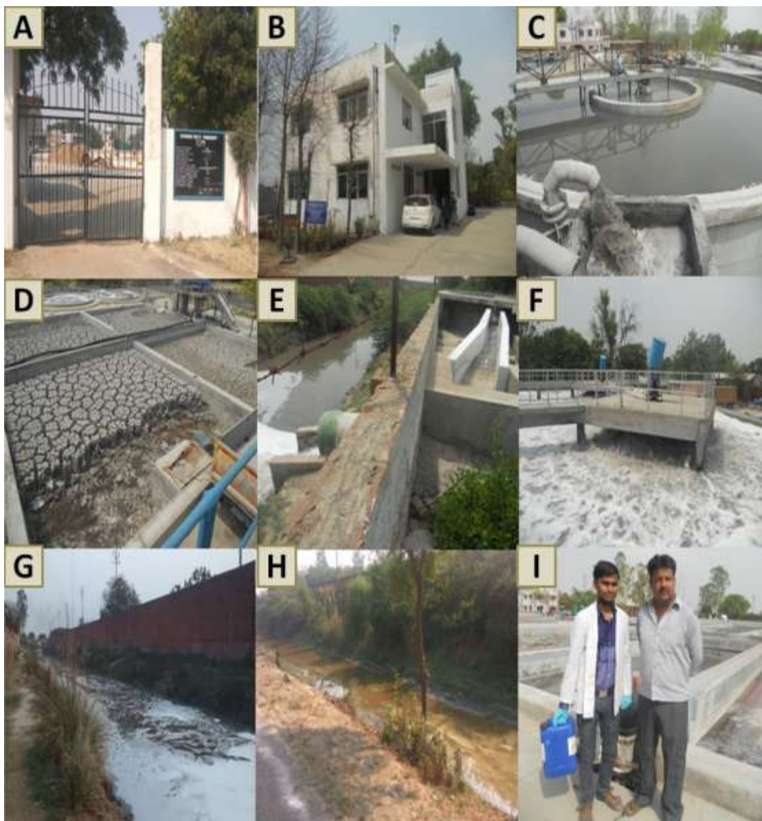
Fig. 4.2 Pics showing TWW treatment, discharge and its collection as well as sludge generation from CETP (A - I)
