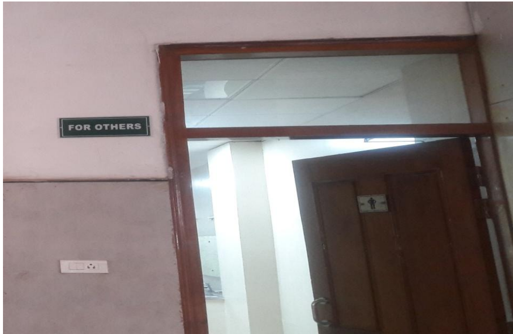
Picture no. 4.1: Washroom constructed for third genders in High Court of Lucknow
