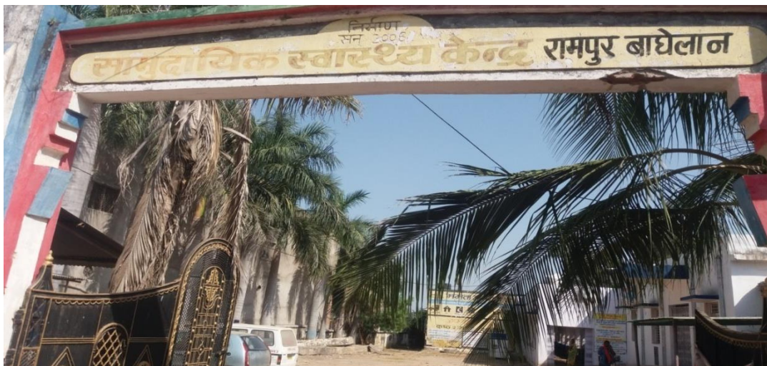
3.19 Image of Rampur Baghelan CHC
