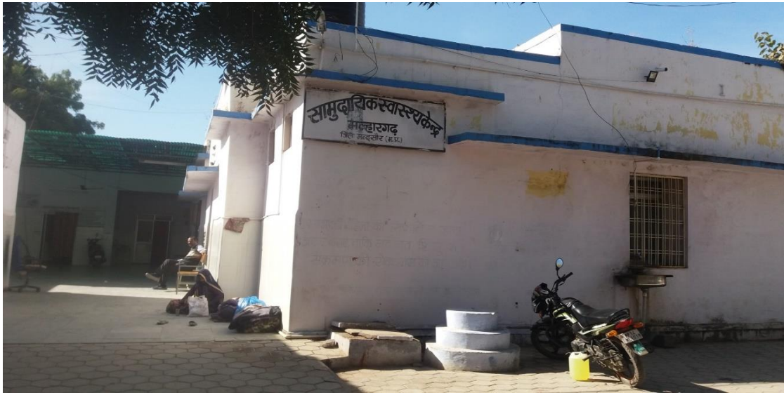
3.23 Image of Malhargarh CHC
