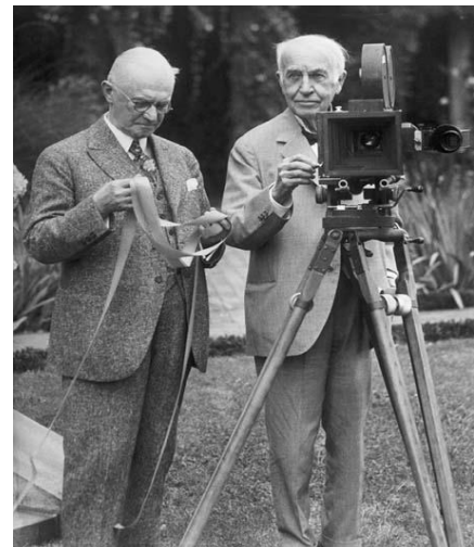
Figure 1: Thomas Edison (right) demonstrates the kinetograph, motion picture camera, with George Eastman, who helped to develop the film used in early motion picture machines.
