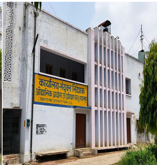
Figure 7: Side view of Main Office
