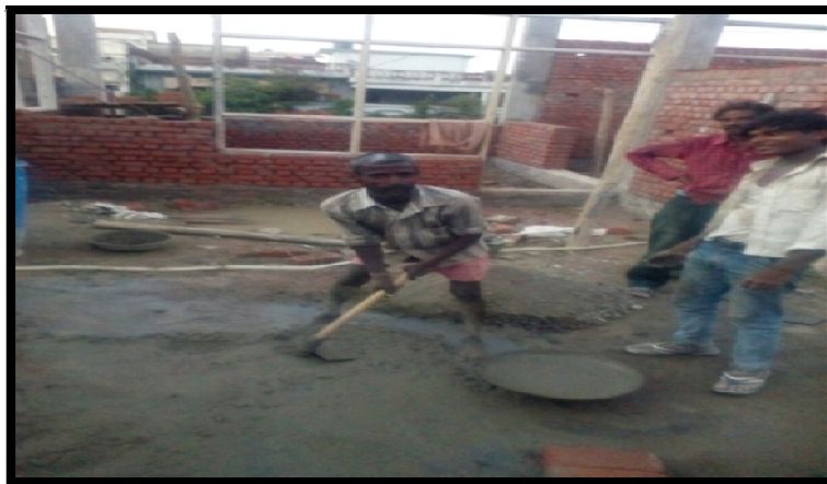
Fig. No. 3.1 Construction workers in site
